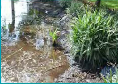
Shoreline erosion due to wave action.
