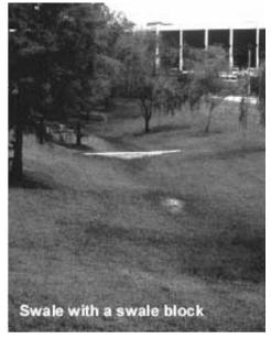
Ponding of runoff in the swale allows the water to soak into the soil, helping to reduce the volume and amount of pollutants.
