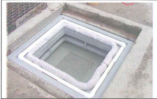
After installing drop box insert and before grate put back on
