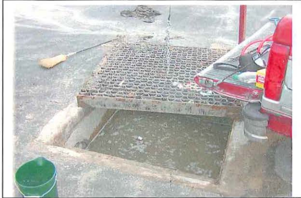
Before installing drop box insert With protective grate partially remove
